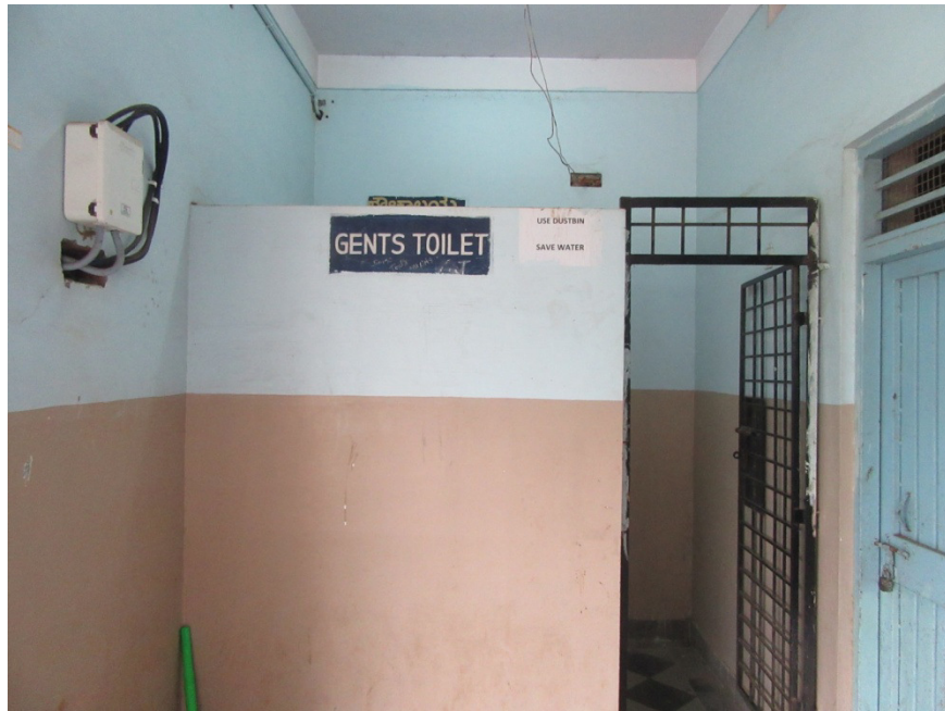
BOYS WASH ROOM
